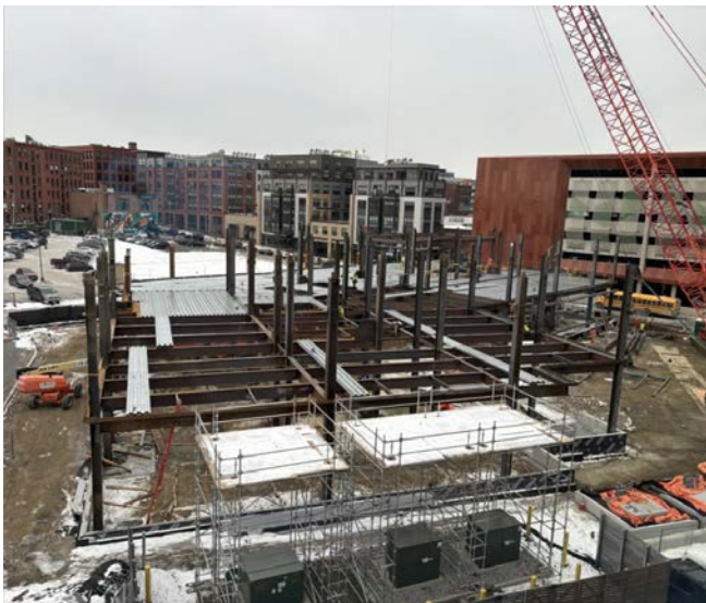
Figure 2. Construction of 150 Richmond
