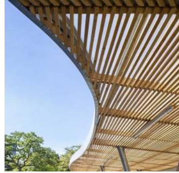
COMPOSITE WOOD TRELLIS AND CEILINGS OF BALCONIES
