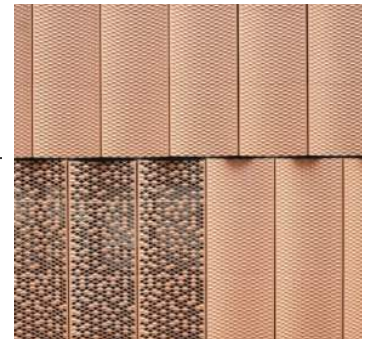
CONCAVE BRONZE PERFORATED AND SOLID METAL PANELS
