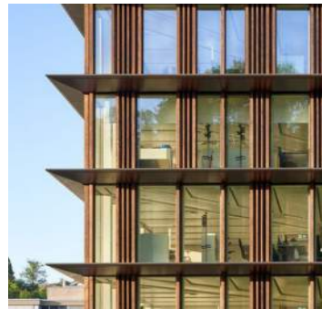
RESYSTA WOOD SCREEN AND FLOOR-TO-CEILING STOREFRONT
