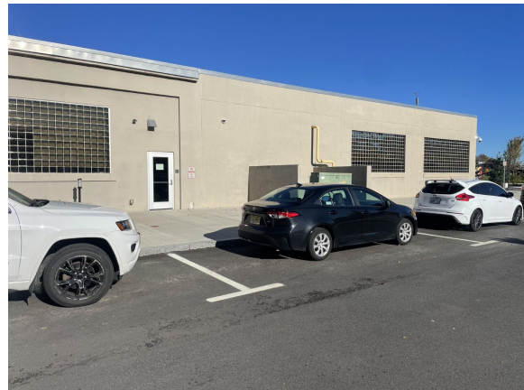
Figure 25 Unregulated Segment of Dorrance Street
