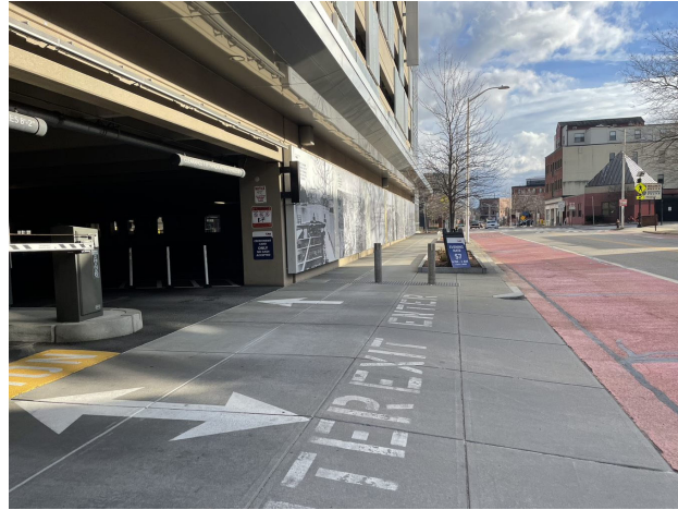
Figure 17 SSL Garage Entrance
