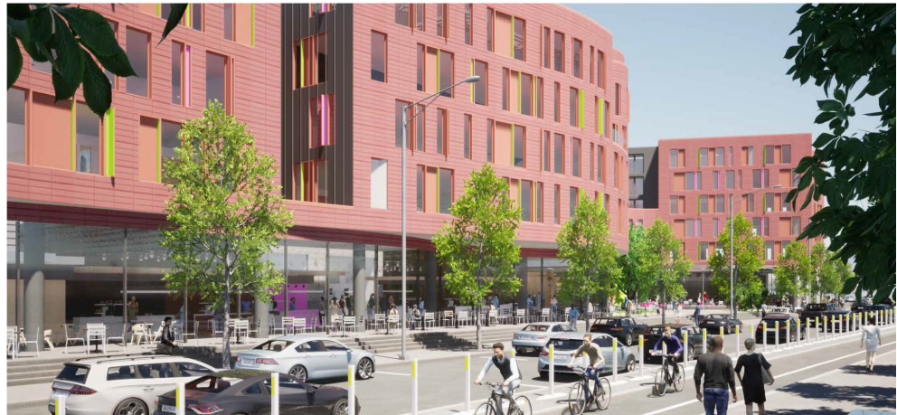
Revised: South Water Street Looking Southeast
