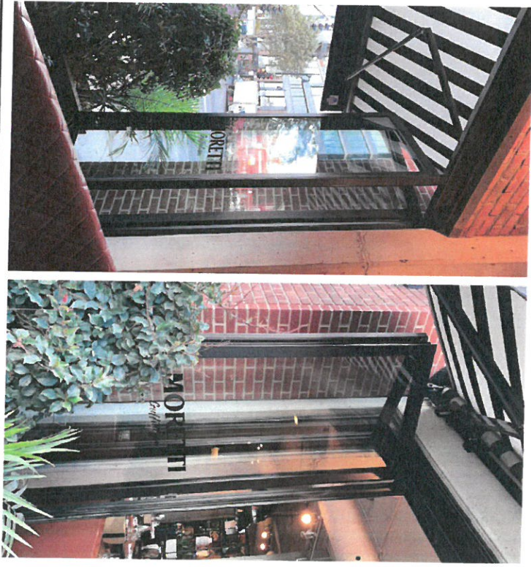
INWARD FOLDING WALL DETAIL GROUND FLOOR
