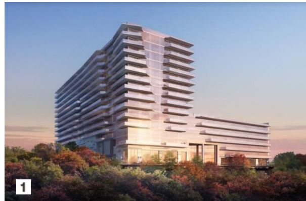
1 One Park Condos Cliffside Park, NJ Luxury condominium ground up development project, DMG in-house management project Gross 417,045-sf, 204 condo units
