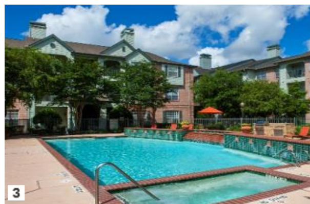
3 Auden Houston Houston, TX Renovation and DMG in-house management project., Gross 202,582sf, 322-bed student housing
