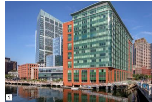
1 Independence Wharf Boston, MA Renovation and repositioning of 470 Atlantic Avenue along Boston’s Fort Point Channel.
