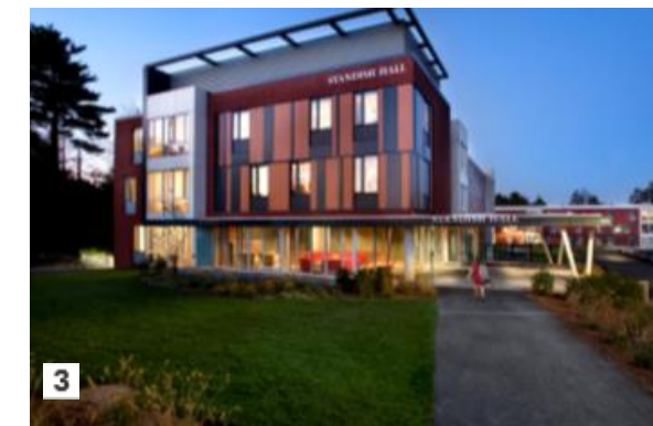
3 Endicott College New Residence Hall Beverly, MA New 62,000-sf, 250-bed student residence hall
